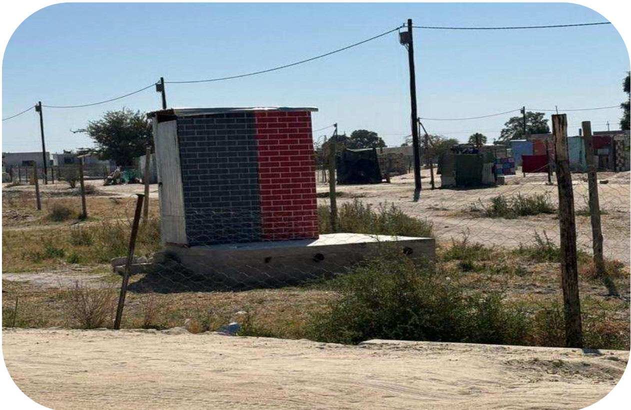
Figure 6: Existing On-site Pit Latrines and Electrical Network
