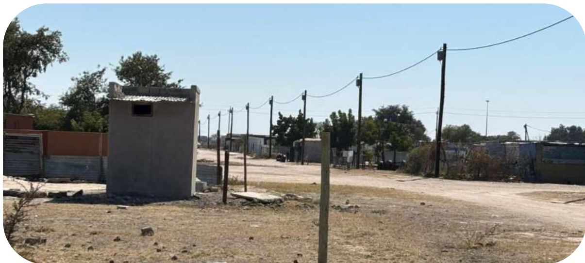
Figure 6: Electricity Lines and Pit Latrines
