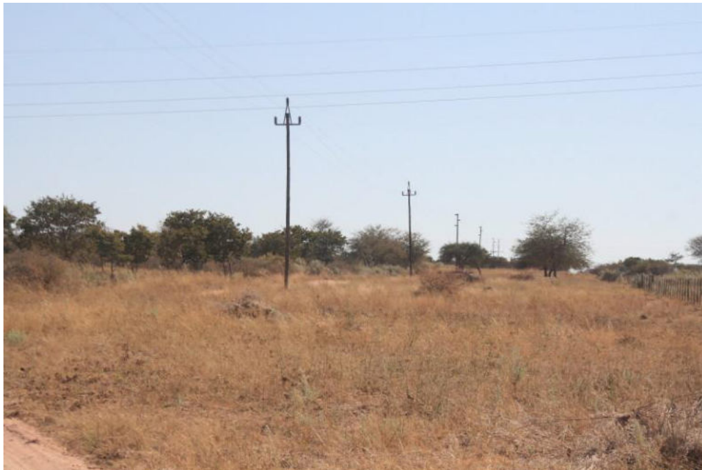
Figure 2. Large sections along this line have been cleared although there are dense patches of Terminalia sericea .
