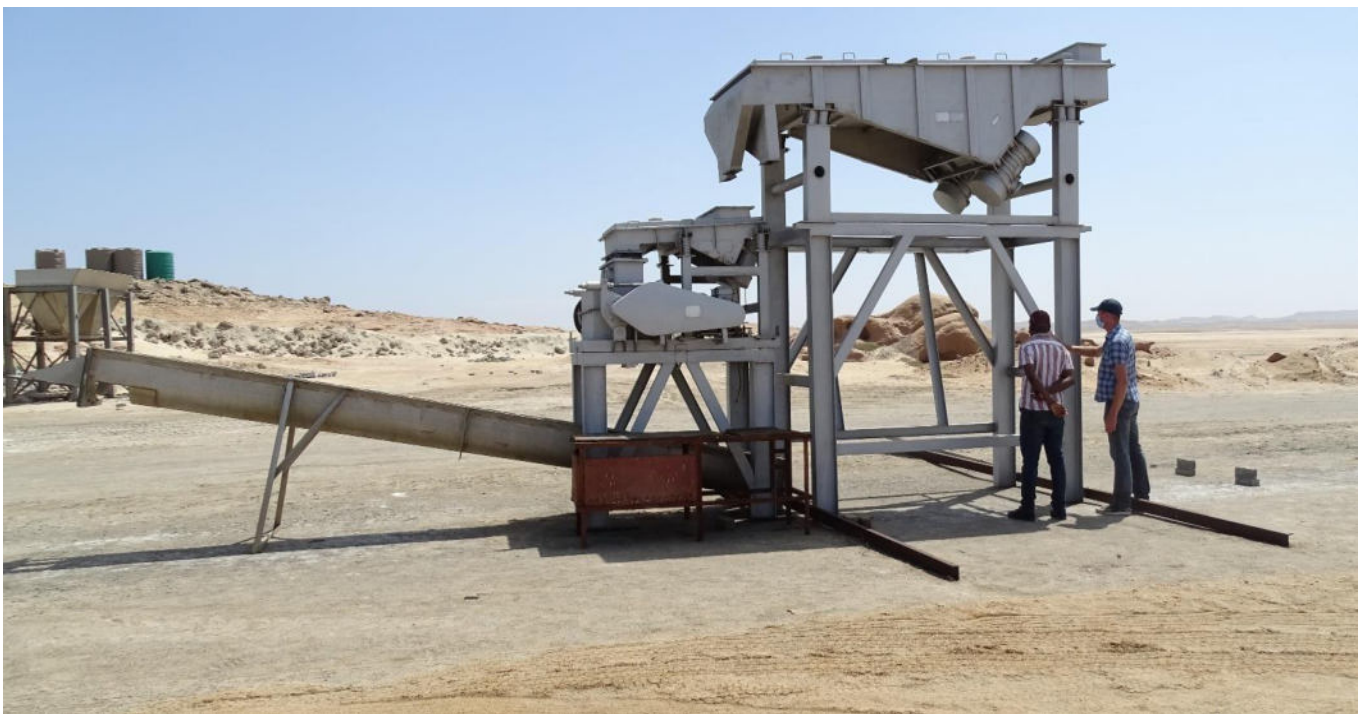
Photo 17: Refurbished coarse salt processing hopper.
