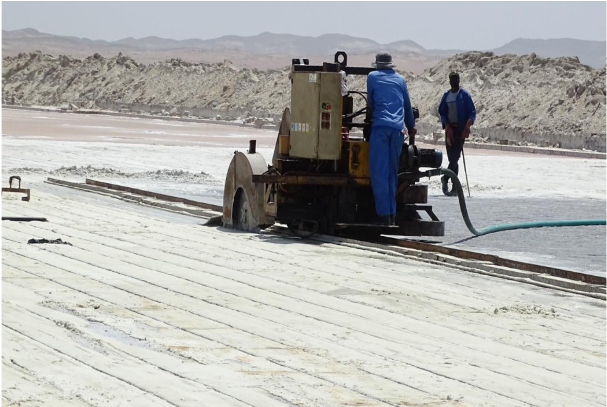
Photo 9 , Some employees employed to operate salt stripping machines with circular blades on site.
