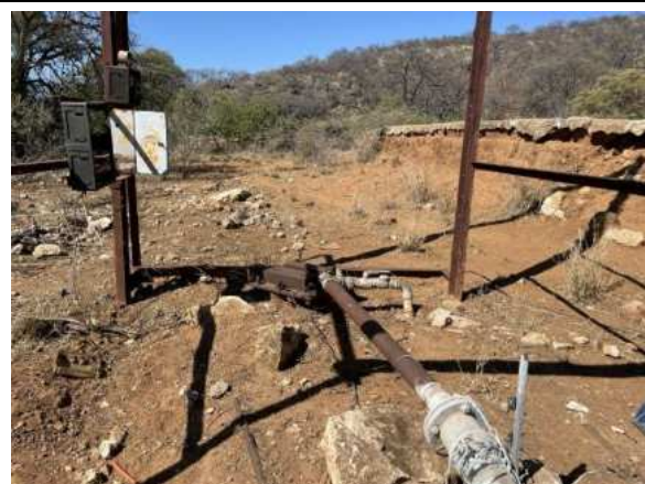
Photo 4-46 EB7 Not used/dry boreholes
