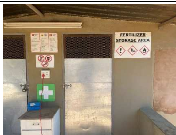
Photo 4-28 Fertilizer storage room entrance
