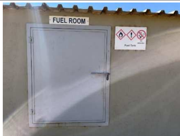
Photo 4-24 Fuel storage room
