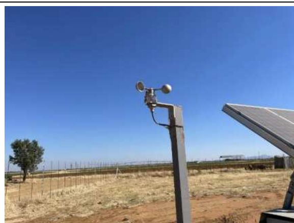
Photo 7-2 Small weather station installation
