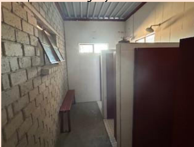
Correct mosaic tiles slope, plaster walls
