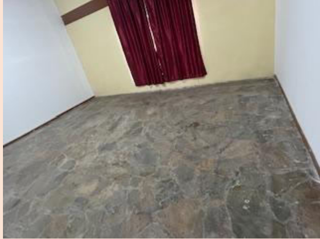
Hostel rooms: rough tiles
