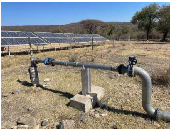
Photo 4-25 BH4 Irrigation borehole WW200927
