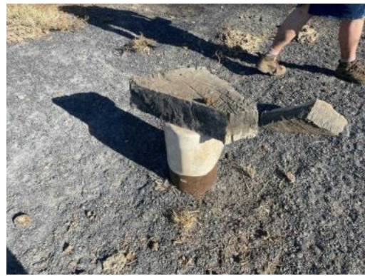
Photo 7-10 EB10 Not in use/dry
