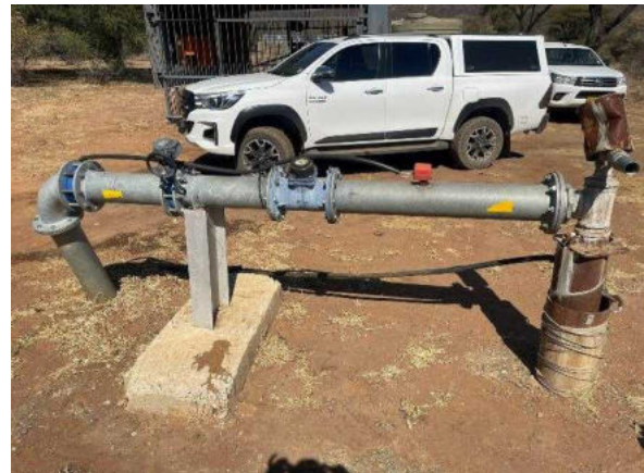
Photo 4-24 BH2 Irrigation borehole WW200925
