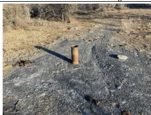
Photo 7-6 EB6 - Not in use
