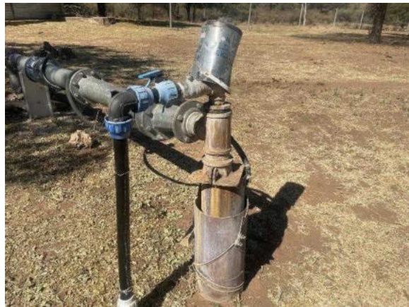
Photo 4-23 BH1 Irrigation borehole
