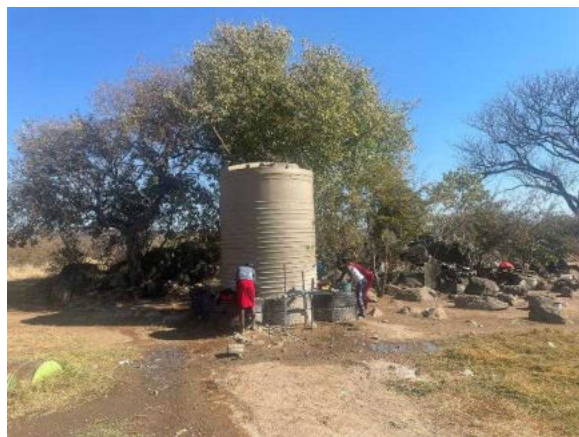
Photo 4-17 Domestic water storage tank
