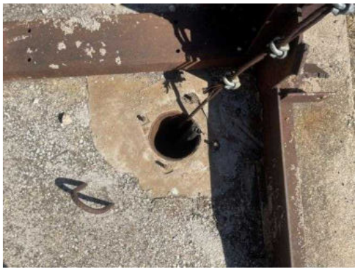
Photo 7-9 EB9 Not in use/dry
