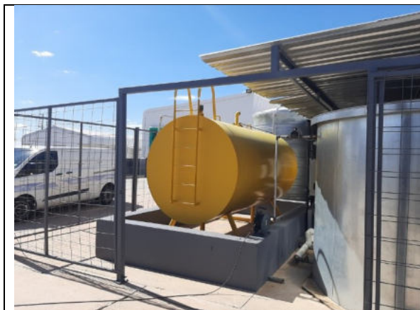
Photo 3-11 Existing diesel tank
