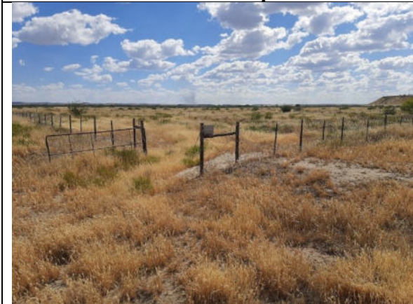
Photo 3-17 A section of the landfill area
