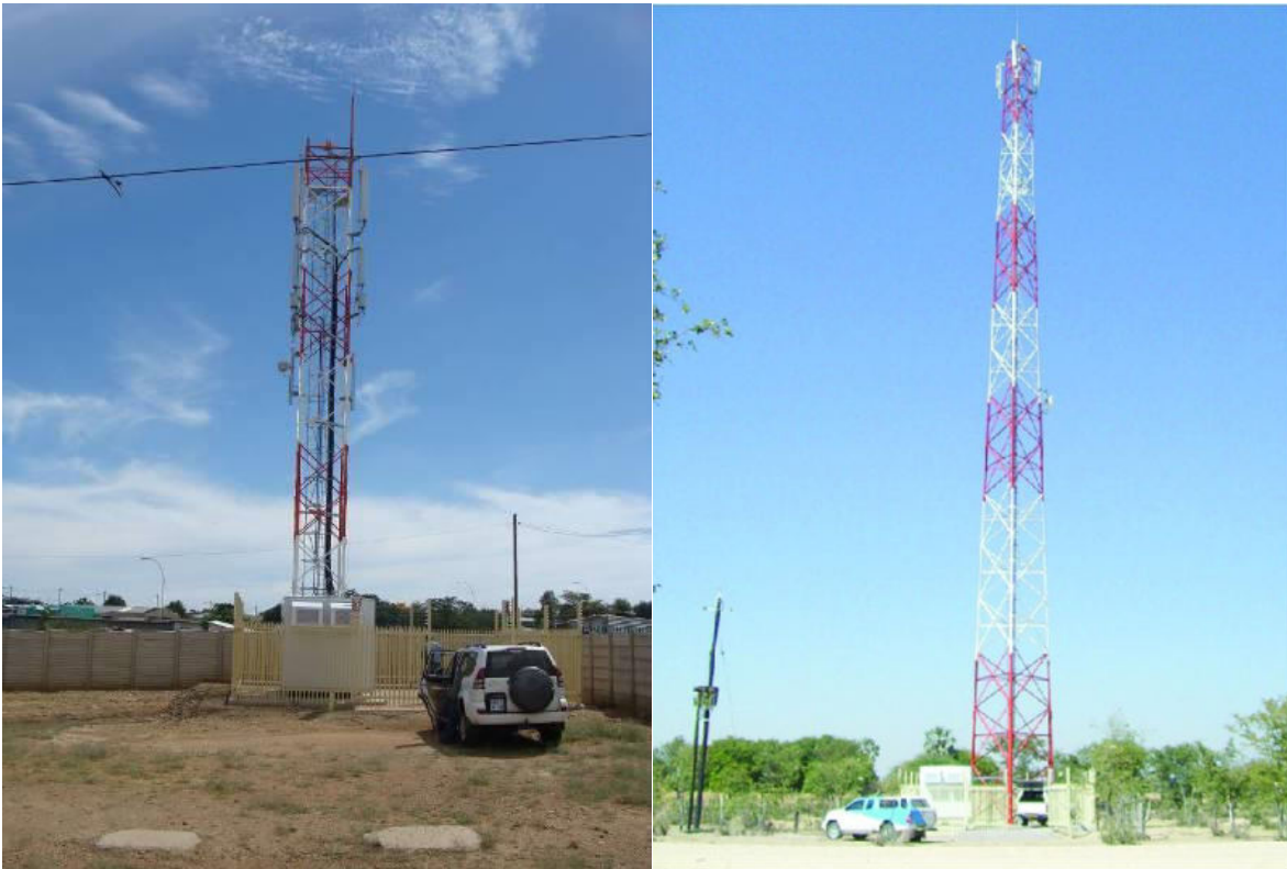
Figure 2-1: Typical red and white painted lattice tower structures in Namibia (source: MTC Namibia and The Namibian newspaper, 2024)
