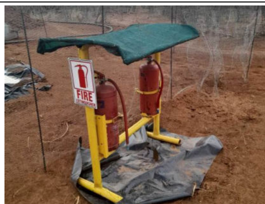
Photo 4-10 Firefighting equipment at drill site
