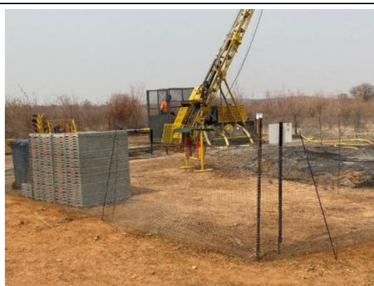
Photo 4-7 Core drilling site
