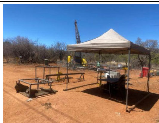
Photo 4-8 Core drilling site
