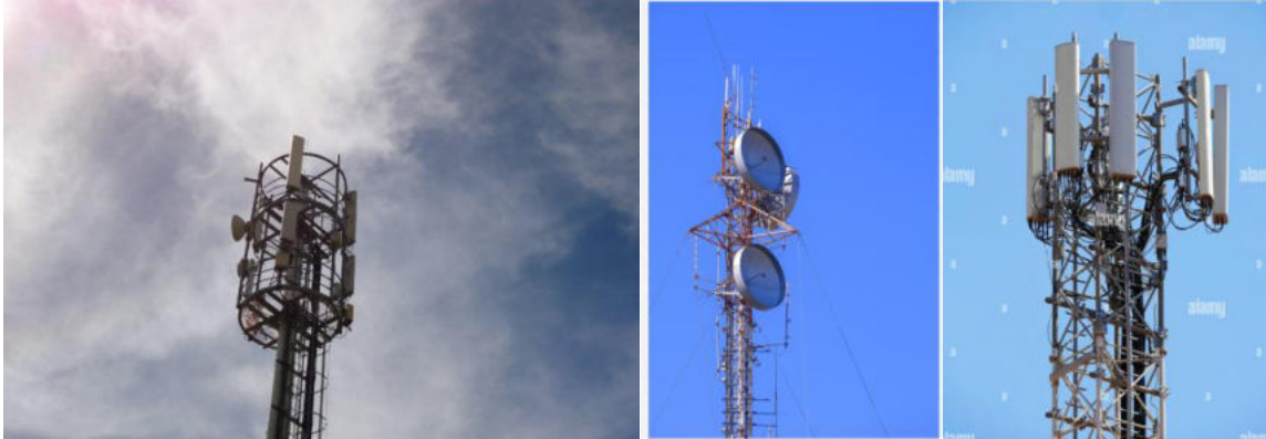
Figure 2-2: Different types of panel-type antennae
