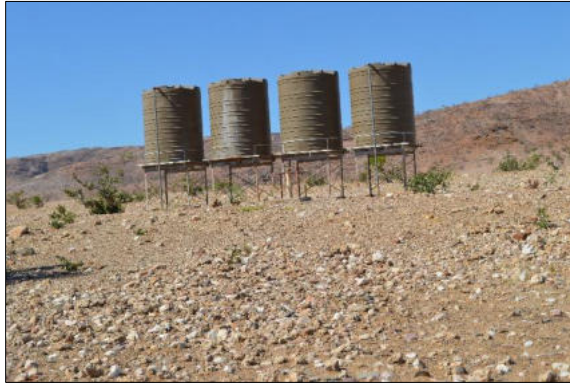
Figure 5-12: Some of the water tanks in the Marienfluss Conservancy
