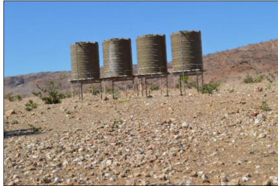
Figure 5-14: Some of the water tanks in the Marienfluss Conservancy
