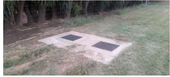
Photo 4-14 Septic tank and soak away on site
