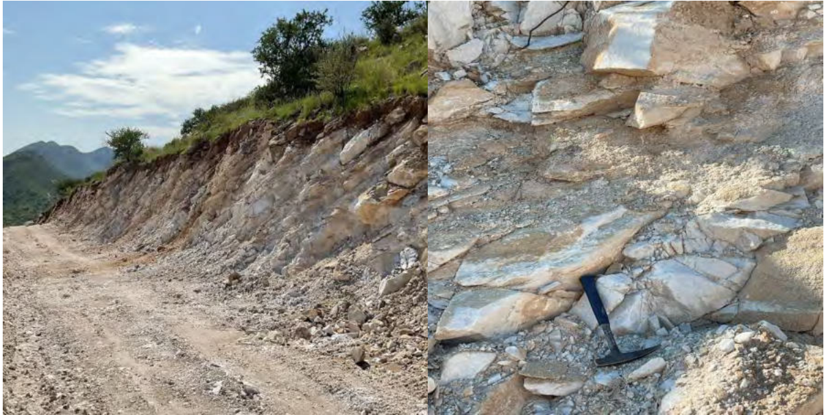
Figure 5-1: A stripped area within the ML 271 with exposed deposit of targeted white marble resources.
