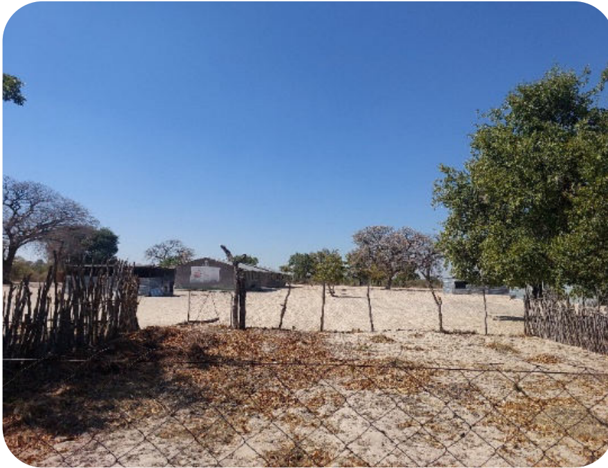
Figure 2-5: Okanaimbula Primary School (Source: Wana Engineering Consulting, 2025)
