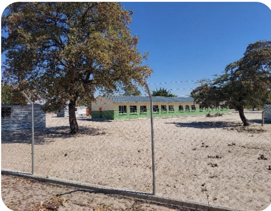
Figure 2-6: Omishe Combined School (Source: Wana Engineering Consulting, 2025)
