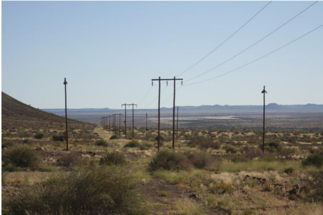
Figure 3. The line passes some hills and rocky terrain northeast of the Naute Dam Substation. See the “dummy” poles to lure sociable weavers making nests on the distribution poles.
