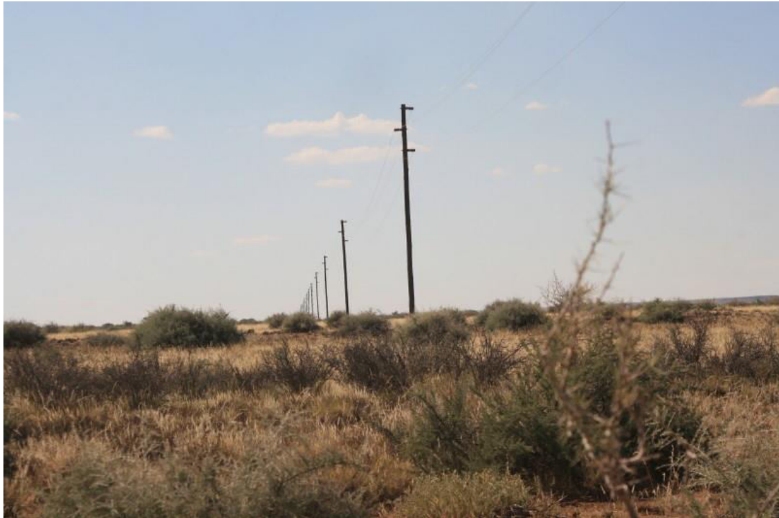
Figure 2: The 22kV Harib – Schonau distribution line with wooden structures.
