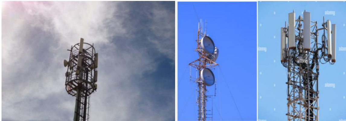
Figure 2-2: Different types of panel-type antennae
