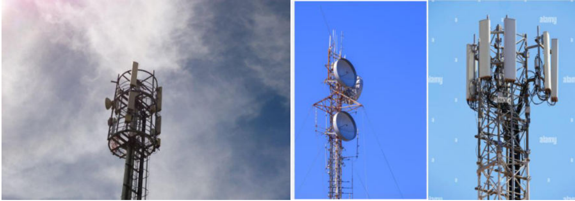
Figure 2-2: Different types of panel-type antennae
