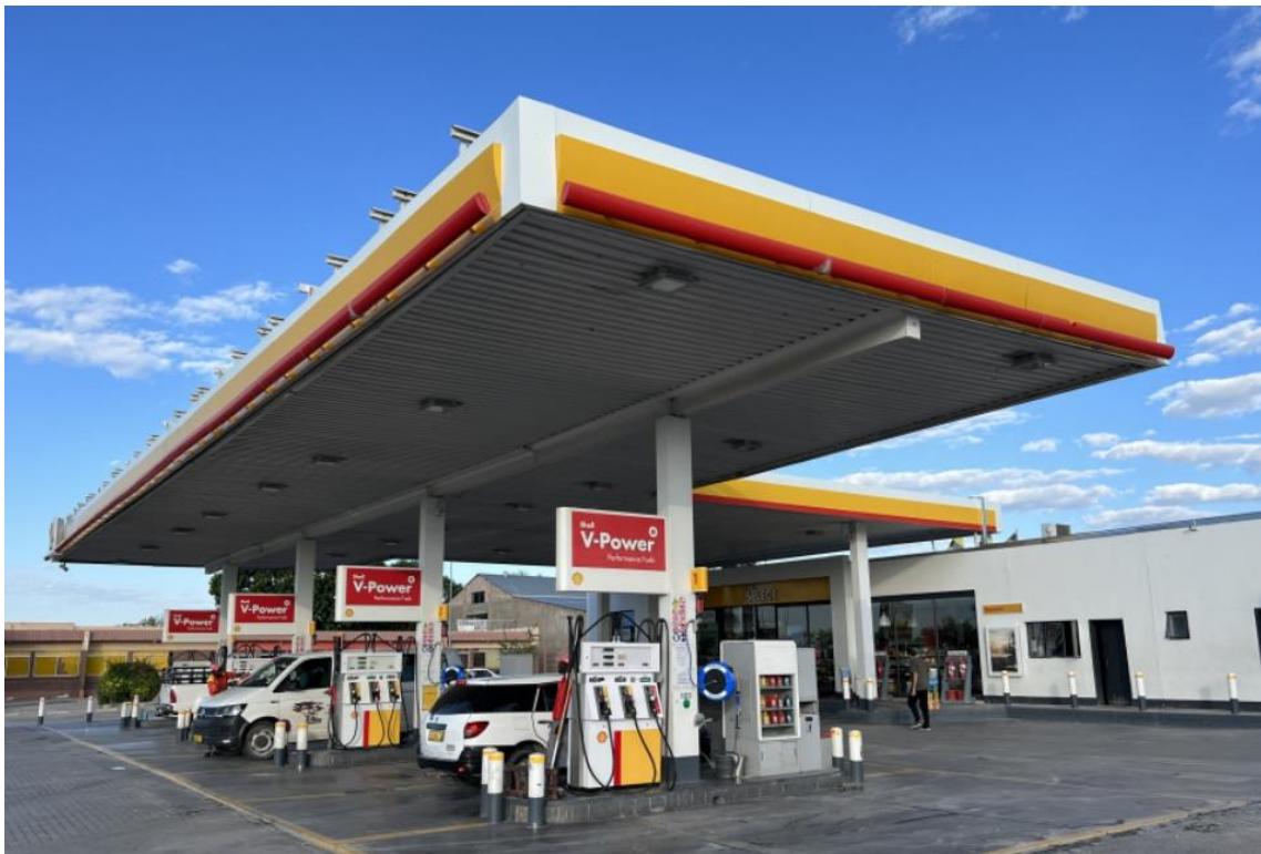
Photo 1. The existing Maroela Motors Service Station .
