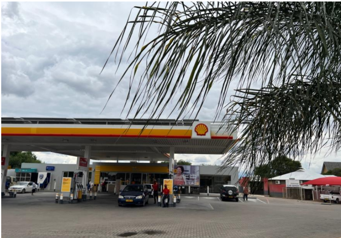
Photo 1. The existing Northgate Service Station .
