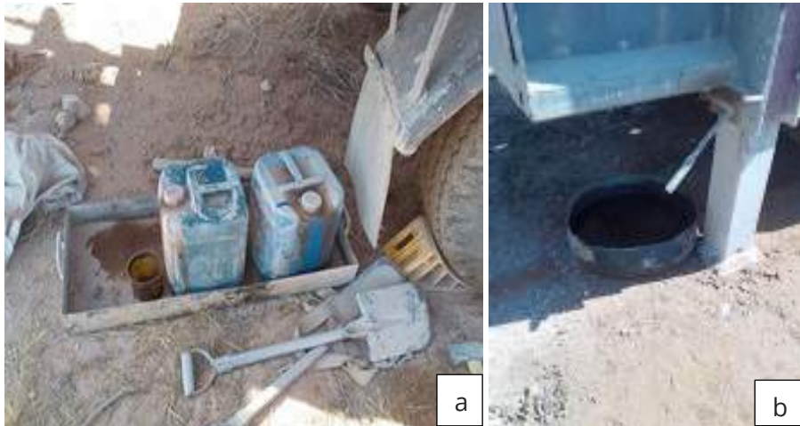
Figure 4 - Hydrocarbon storage (a) and oil containment at drill pad (b)
