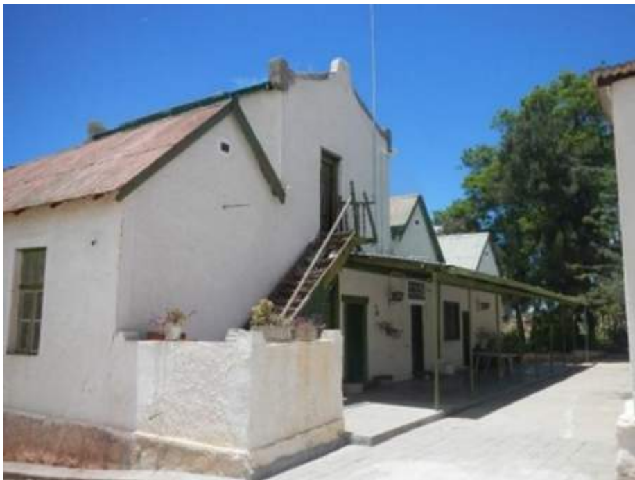
Figure 130 - Back view of the well- constructed historical Okawayo 481 farmstead (Kinahan, 2021).
