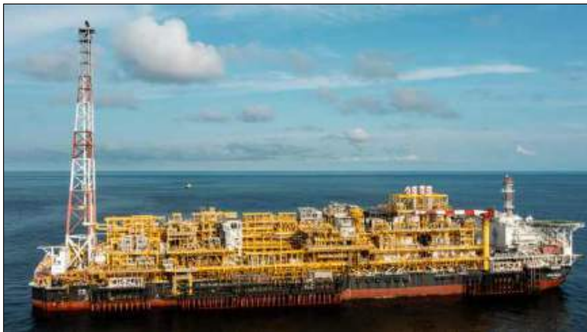
Figure 5-11: Example of an FPSO
