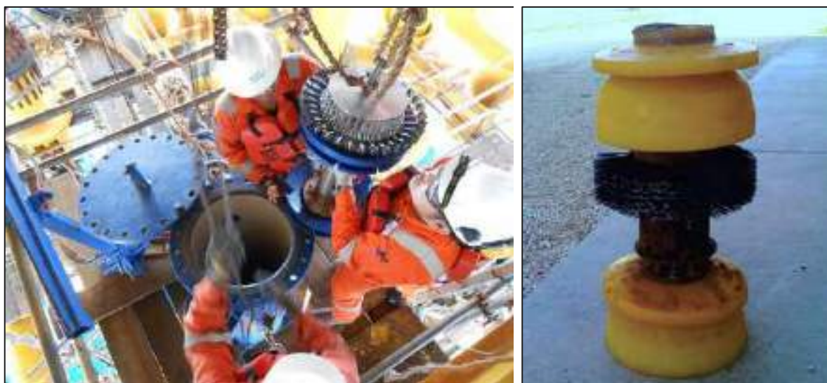
Figure 5-7: Insertion of a “pig” into a pipeline (left) and a wire brush cleaning pig (right)
