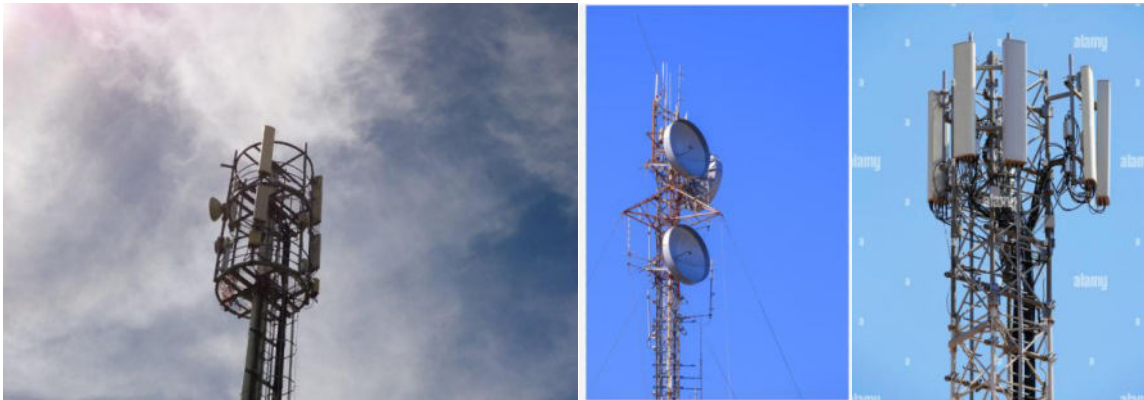
Figure 2-2: Different types of panel-type antennae
