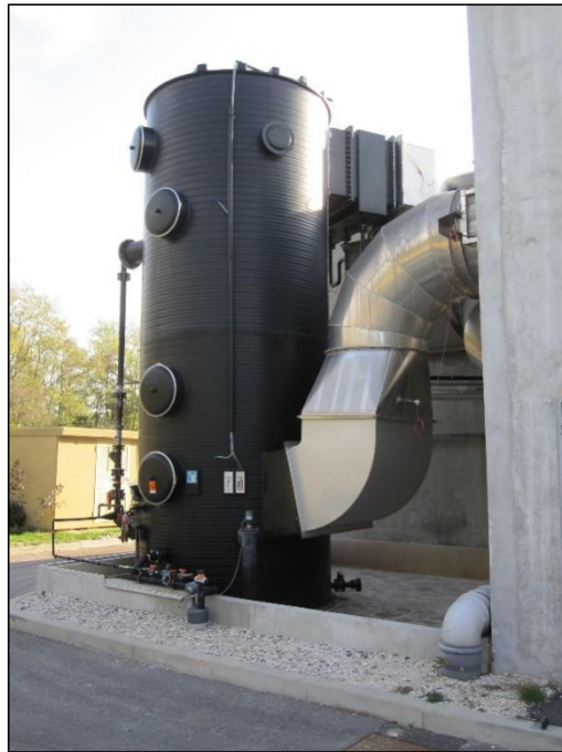
Figure 5: A typical scrubber (air/gas entering via the duct on the right)
