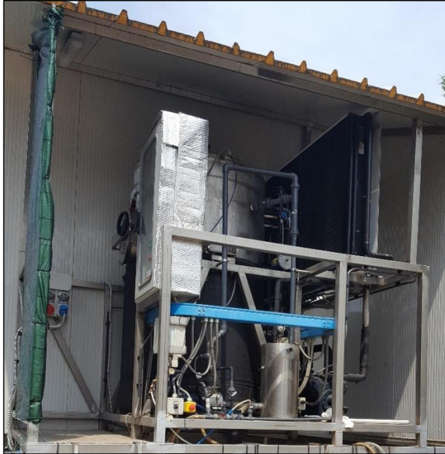
Figure 7: An evaporator-concentrator unit
