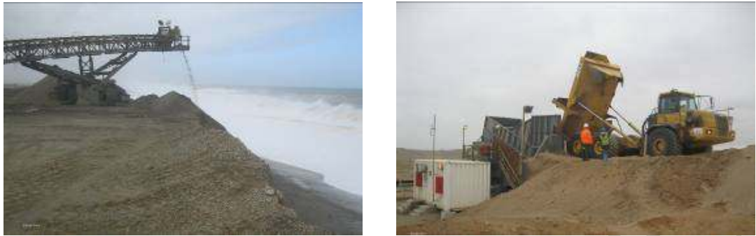
Figure 1. Loading (left) and deposition of overburden material onto the beach with conveyors (right) to achieve accretion.
