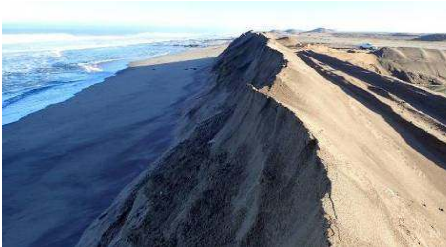
Figure 24. Northern block test mining: Temporary seawall (photo Namdeb).
