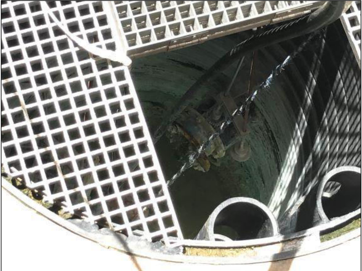
Figure 14-2: Cell 1 outlet pipes into HDPE sump
