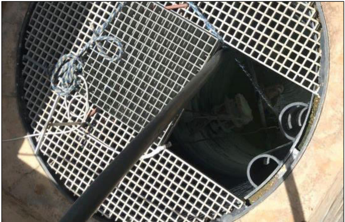
Figure 14-1: Pond 1 pipe outlets into HDPE sump
