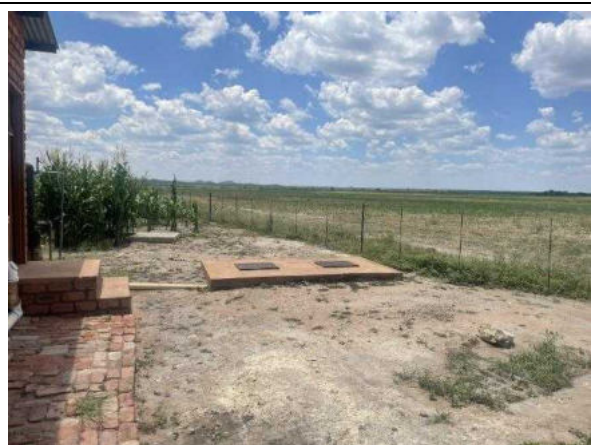
Photo 4-31 Septic tank at worker housing
