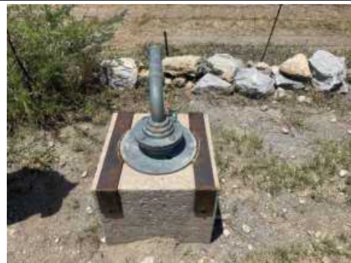
Photo 7-4 BH 4 - Borehole installation for domestic and stock use
