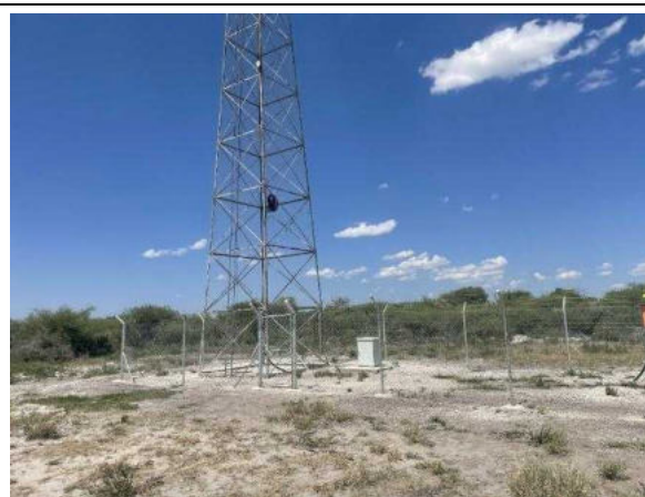
Photo 7-2 Radio mast with lightning conductor
