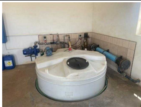
Photo 4-13 Fertiliser mixing tank inside building
