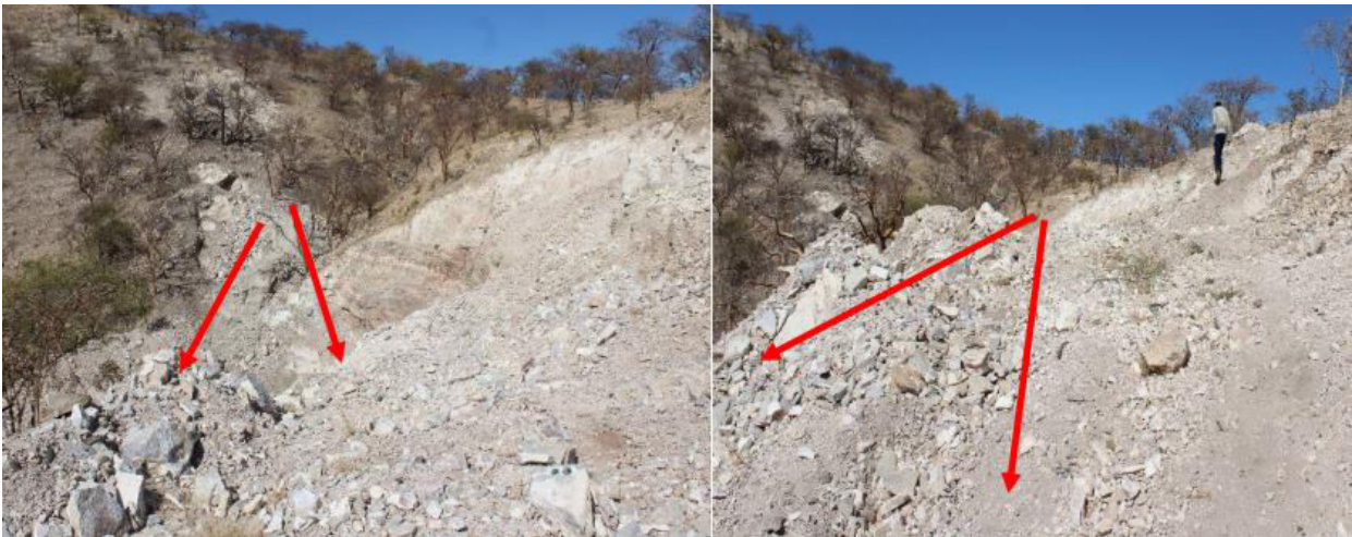
Figure 3: Evidence of trenching on targeted sites
