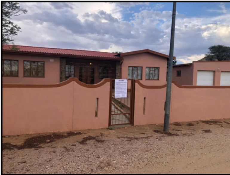
Figure 3, Depicts that are existing structures on the property.
