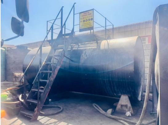
Figure 7:Second tank which will require a bunded wall
