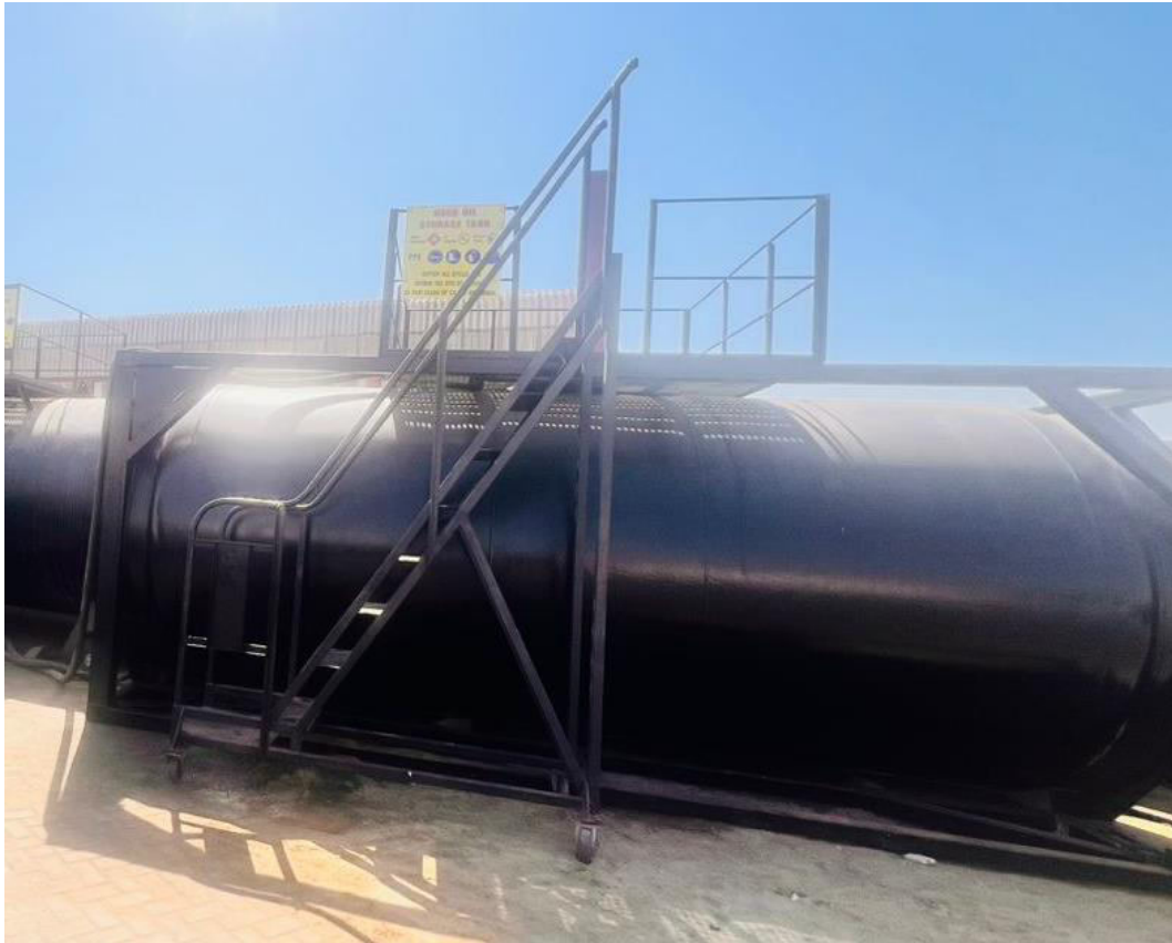
Figure 3: a self-bund tank contained inside a concrete bund
