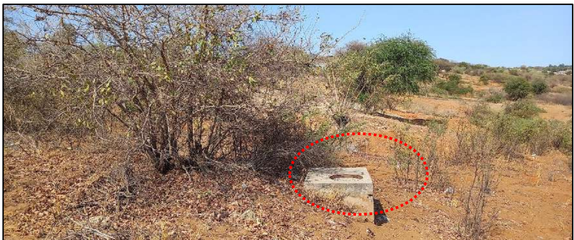
Figure 9: Sewage Inspection Manhole South of Erf 1527
