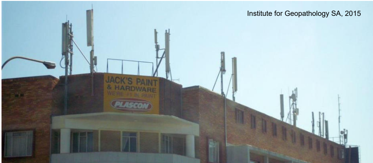
Figure 5-9: Example roof top BTS
