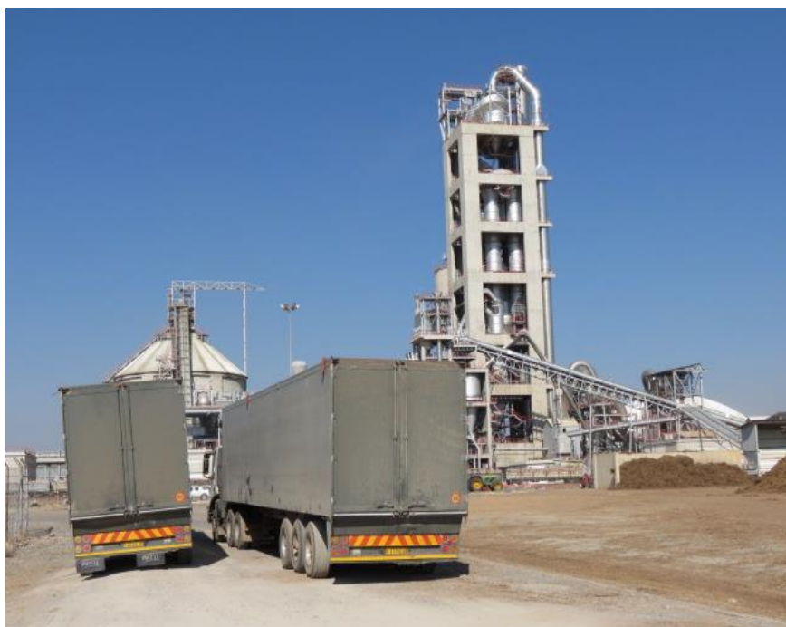
Figure 26: 2 x 110 m 3 biomass transport trucks at Ohorongo Cement
