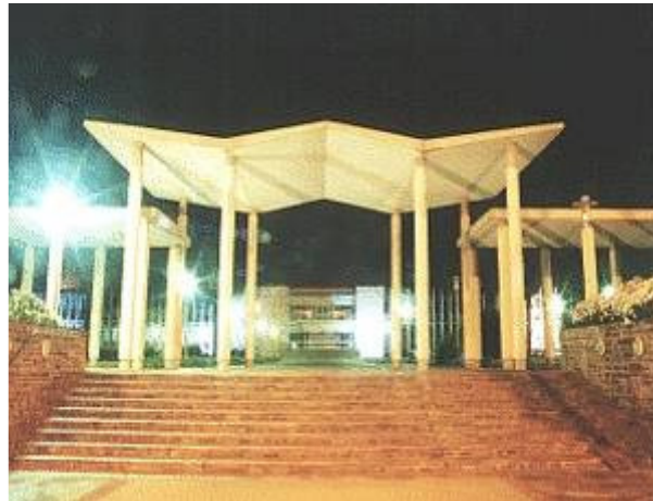
Walvis Bay Civic Centre (Municipal Head Offices)
