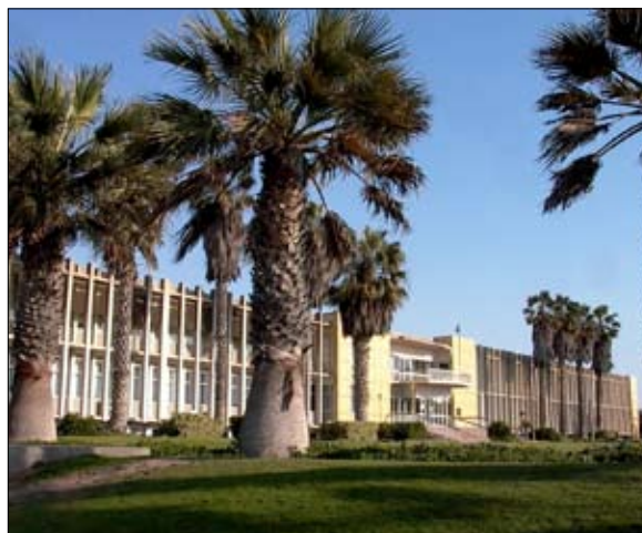
Walvis Bay Civic Centre (Municipal Head Office)
