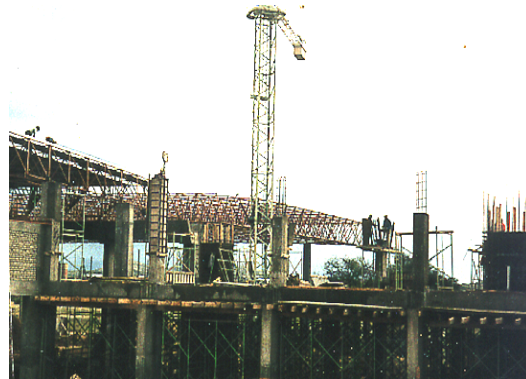
Construction of the Brew house 1985
