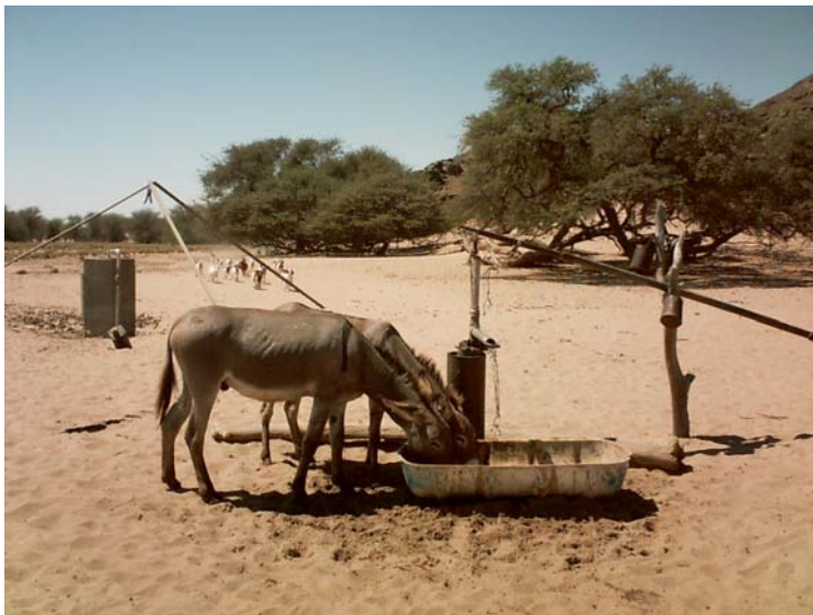
Figure 16: Swartbank , old well point with hand pump and the new borehole
