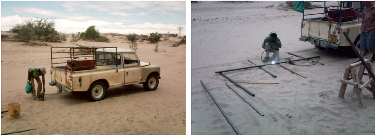
Figure 7: Welding of drill pipes
