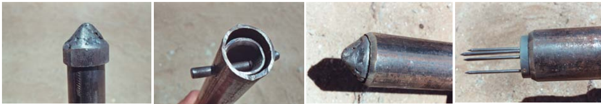
Figure 8: Drilling Pipes for the insertion of the Theta-Probes
