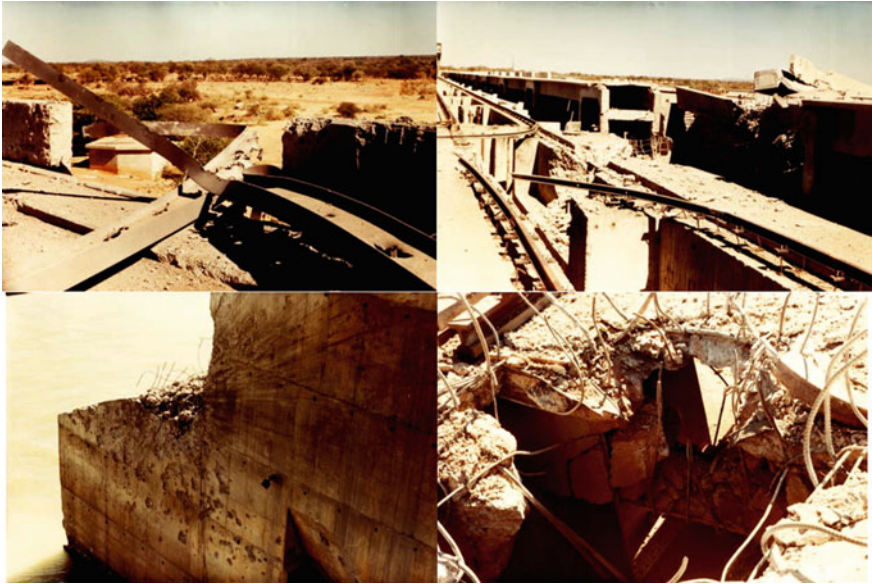
Fig. 2.3 Damage to the Calueque Barrage, June 1988
