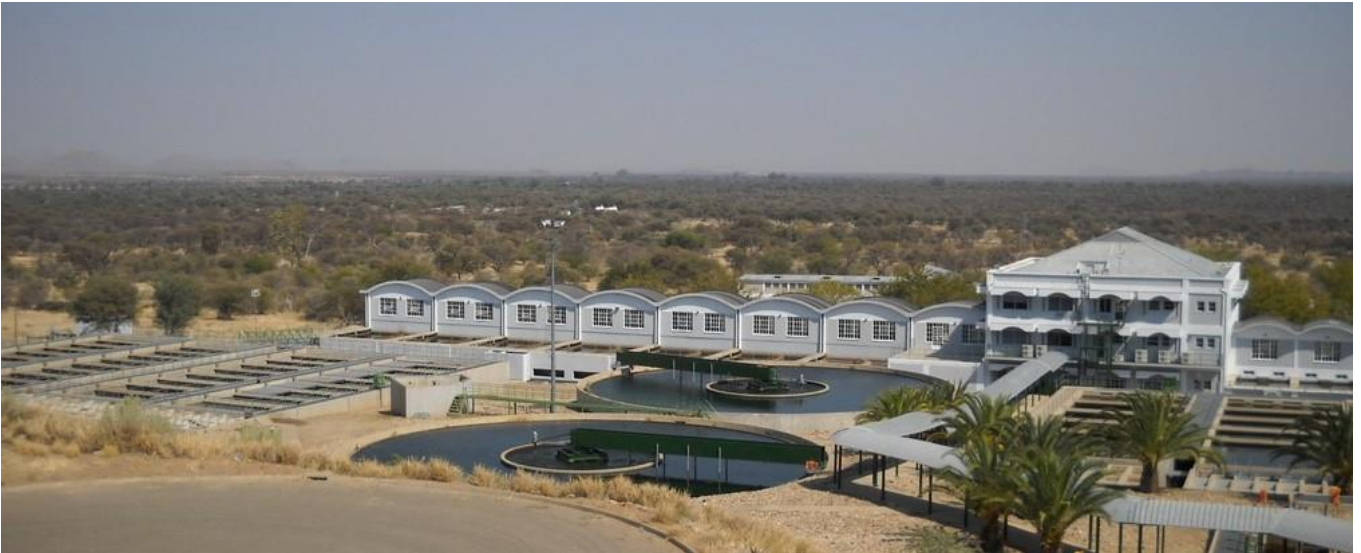
Figure 20: Von Bach Water Treatment Plant
