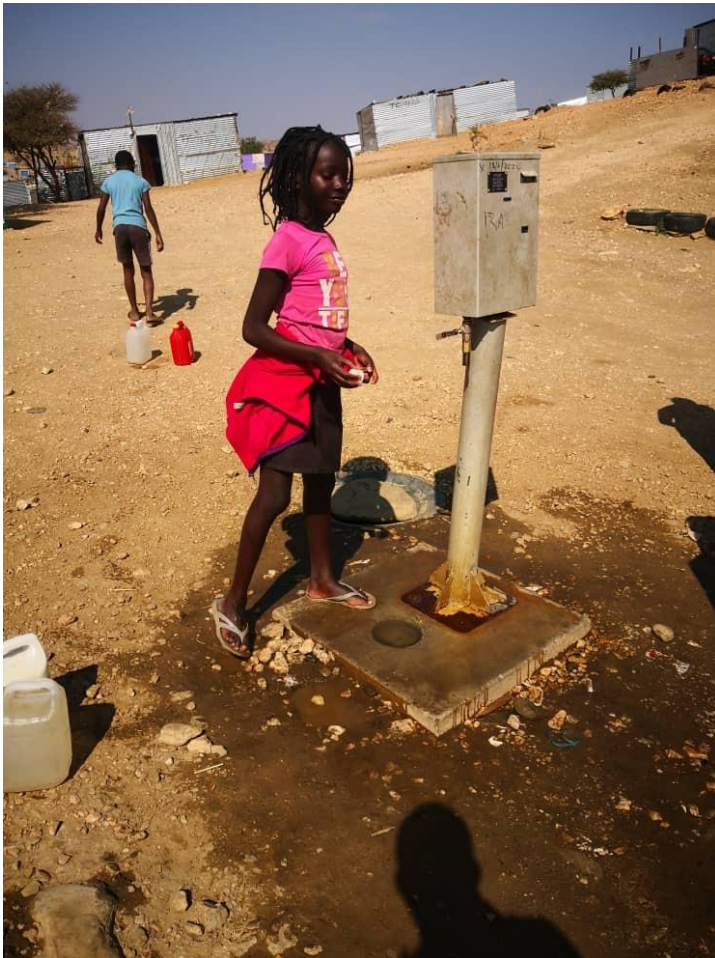
Figure 17: Prepaid Communal Water: Demand Management through emphasis on the value of water
