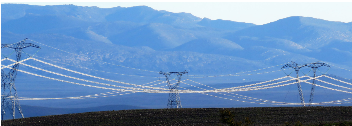
Figure 3: An example of a 400 and a 220 kV power line in parallel with staggered towers showing the greater visibility of the lines with a tower placed opposite the mid span.
