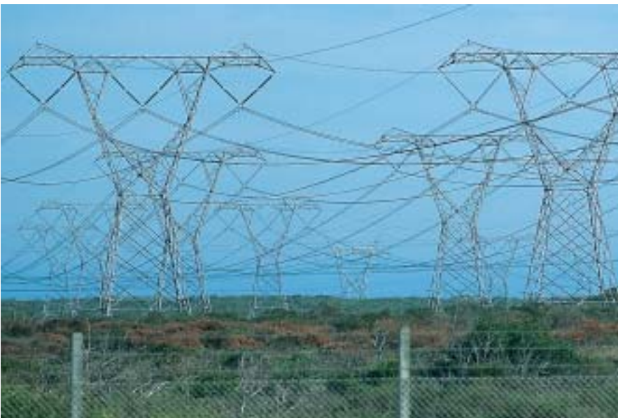
Figure 66. Powerlines crossing strandveld near the Koeberg nuclear power station, outside Cape Town (3318CB).
