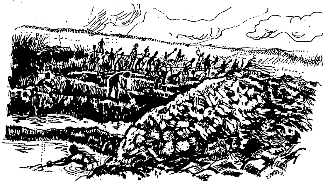
(c) Digging a canal to short - circuit a long river loop.
