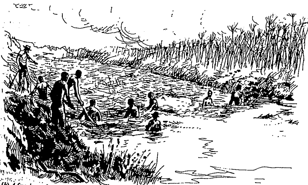
(b) A few days after the initial clearing a secondary obstruction of matted roots etc rises to the surface and has to be removed.
