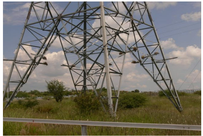
WBSW nests on pylon – Photo : Neil Thomson
