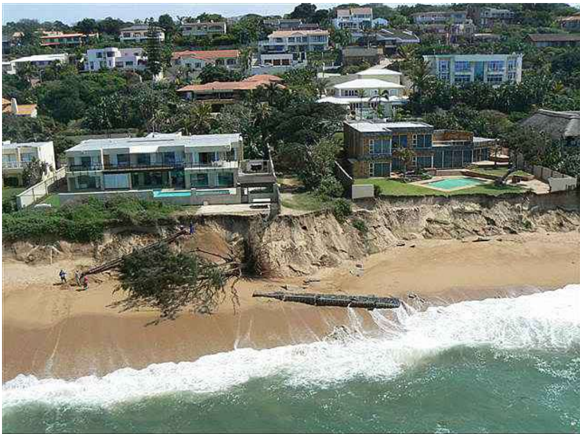
Figure 4: Coastal damage from the March 2006 storm on the KwaZulu Natal, South Africa coast
