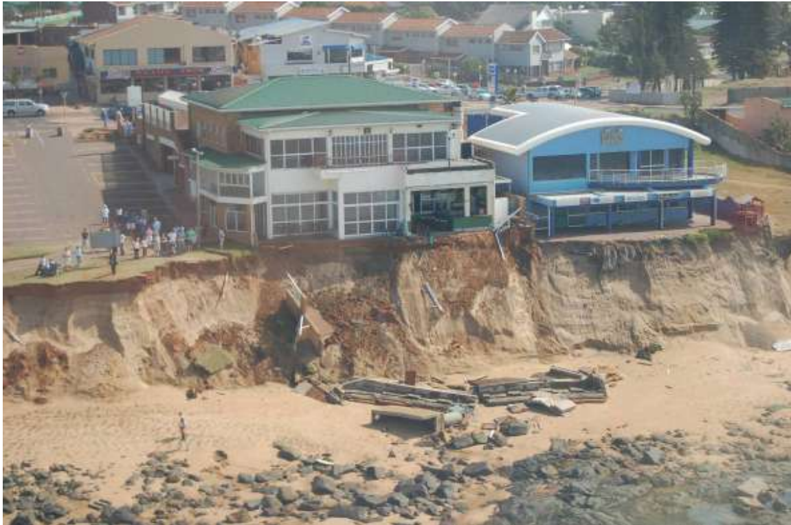
Figure 3: Coastal damage from the March 2006 storm on the KwaZulu Natal, South Africa coast
