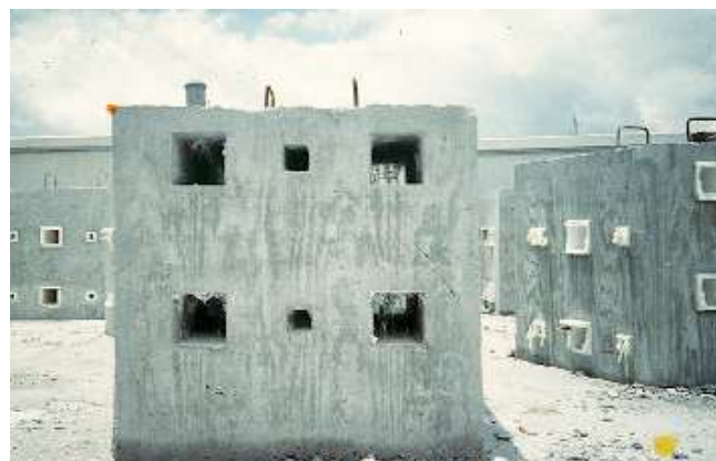
Figure 28: Concrete blocks used off the coast of Australia to create an artificial reef. The rocks have been designed to create refuge for sea-life
