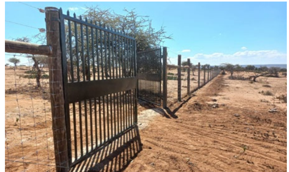
The erection of a 1-kilometer fence at Leberishereki School is ongoing to prevent human-elephant conflict.
