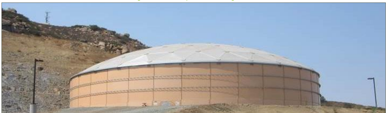
Figure 29: Example of a storage tank
