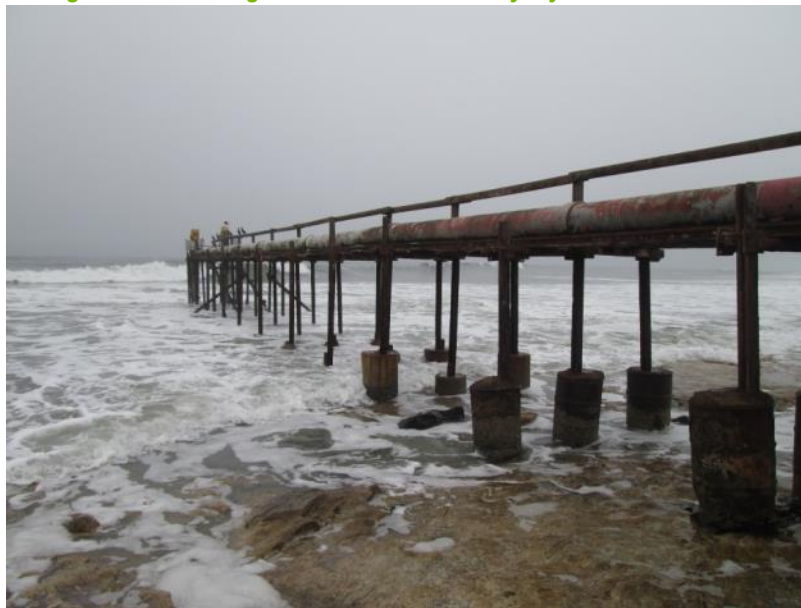
Figure 12: Existing seawater abstraction jetty for the Salt Works
