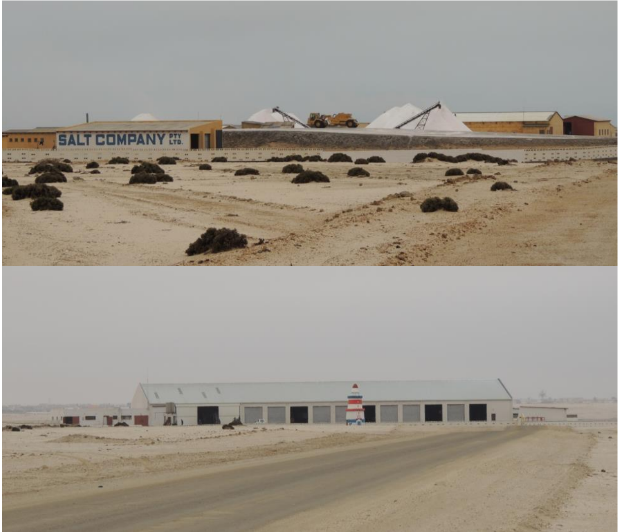
Figure 56: Photograph depicting the existing Salt Company (Pty) Ltd structures and salt stockpiles and warehouse
