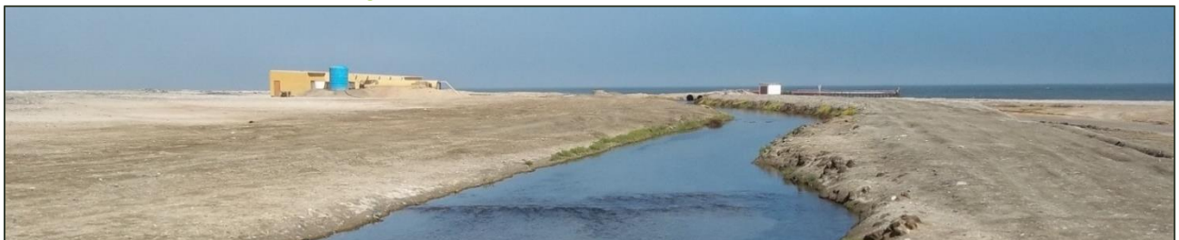
Figure 24: Salt Works Seawater Intake Channel
