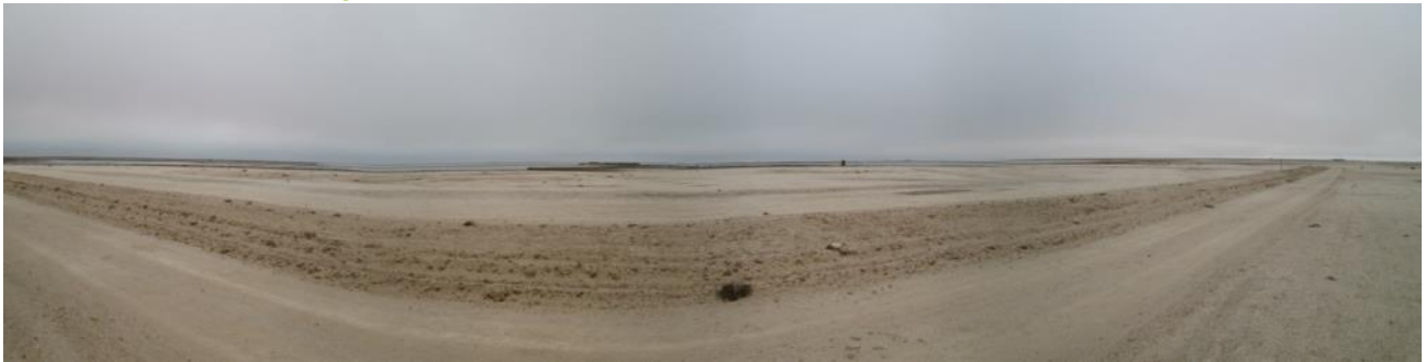
Figure 43: General view of the Base Case desalination plant site
