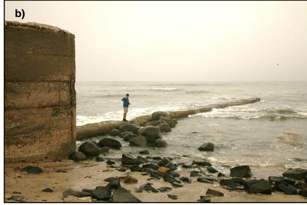
Figure 2.3: a) Rocky shelf at Outfall 5, preferred location; b) Concrete structures at old Saltworks intake – Alternative location - Outfall 1. The old concrete-encased pipe is visible.
